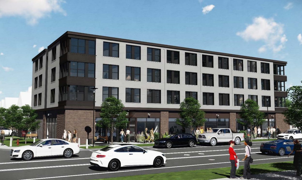
View of the Project looking Northeast from Niagara Street.
