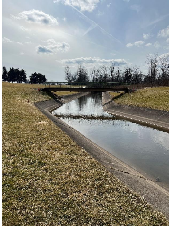
Figure 4: Concrete Channel Downstream of Debris Dam
