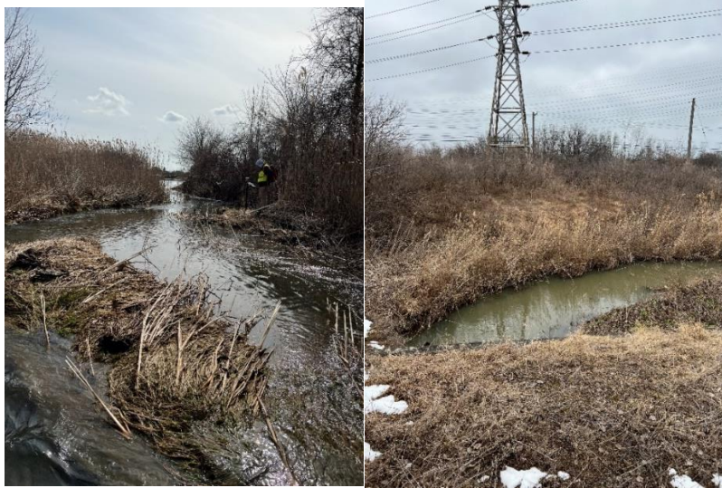
Figure 2: Photos from Upstream of Debris Dam
